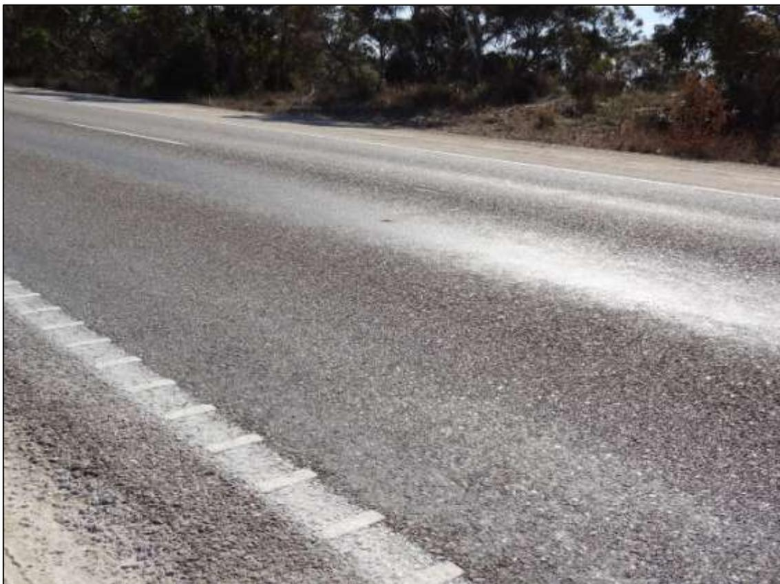
Figure 9 – Severe Rutting and Signs of Aggregate Loss
