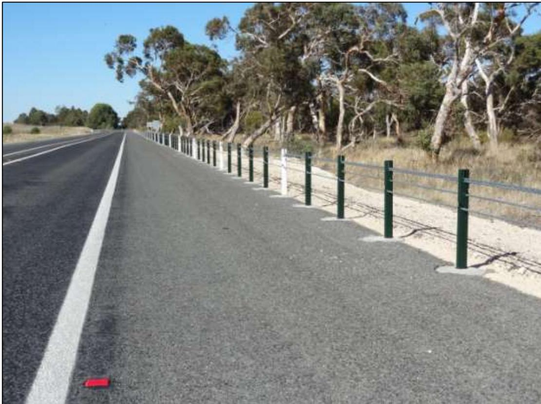
Figure 11 – New Wire Rope Barrier Fencing on the Dukes Highway
