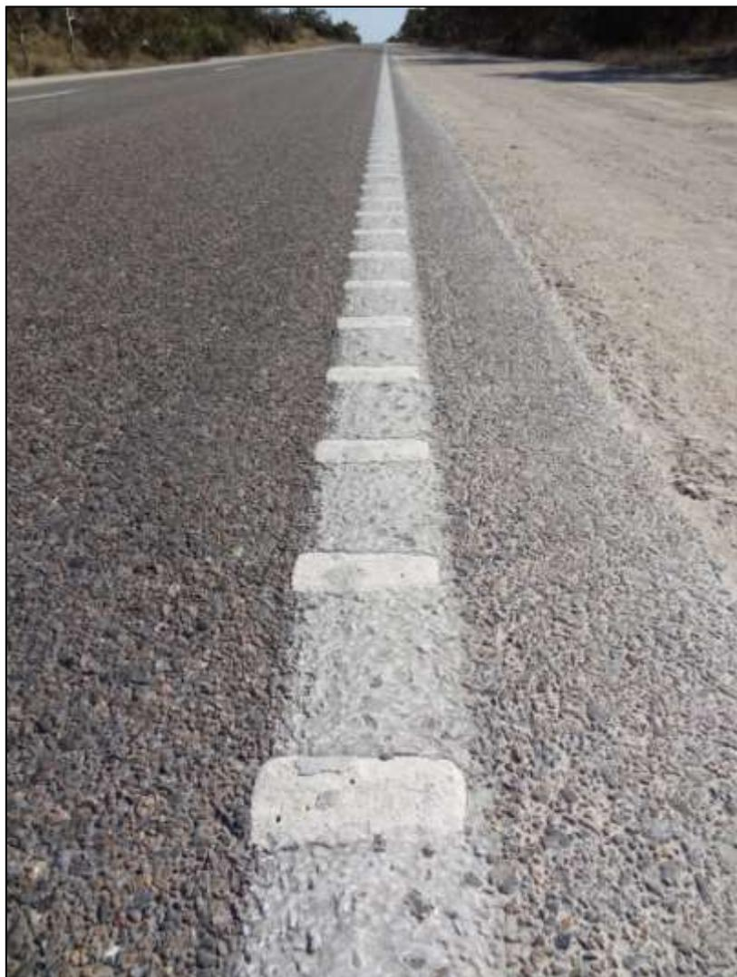
**Figure 5 – Worn Out Audio Tactile Line Markings on the Dukes Highway**
